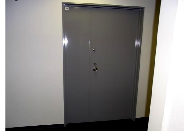
出入口A扉廊下側
