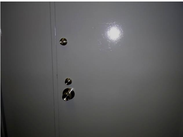
出入口A扉廊下側
